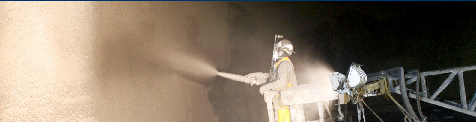
A revolutionary construction process is central to the benefits the Domesilo has over traditional solutions.
