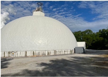
The existing dome was sagging at the apex and had other structural issues, but Dome Technology's evaluation confirmed the structure could be salvaged.
