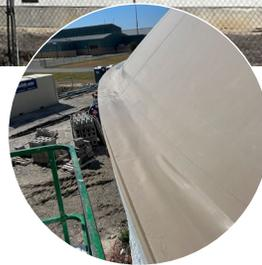
To save money, the customer requested that Dome Technology incorporate factory-produced roof skirting for rain management.
