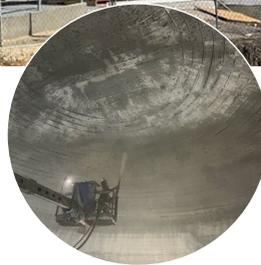
Concrete was applied to the inside of the dome membrane using the shotcrete method.
