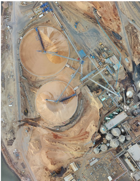
The PCA woodyard now features upgraded circular stackers complete with 2,400 feet of conveyance.
