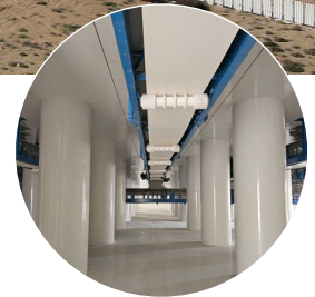
Cleanliness is of utmost importance inside the dome and within conveyance tunnels too, like the one pictured above.
