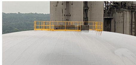
The new reinforced concrete dome replaced a failing steel domed roof.
