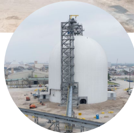
Dome Technology's team fabricated the stair tower and bridge.
