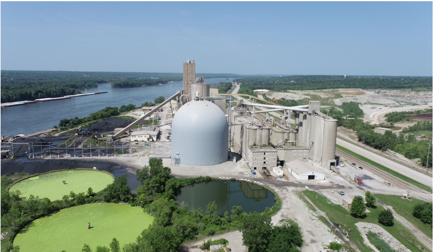
Continental Cement Company's new DomeSilo in Davenport, Iowa, can store 125,000 short tons of cement powder. Cement is reclaimed at 350 stph and pneumatically conveyed to barges on the Mississippi River.
