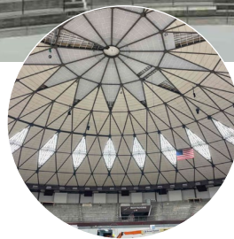
Dome Technology rehabilitated the dome roof, including installation of ceiling tiles.
